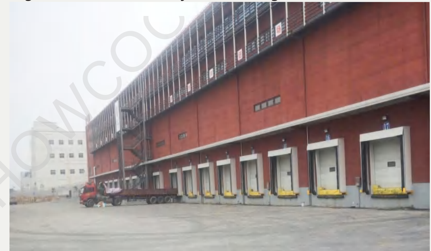
logistics Cold Store Project At Shanghai
