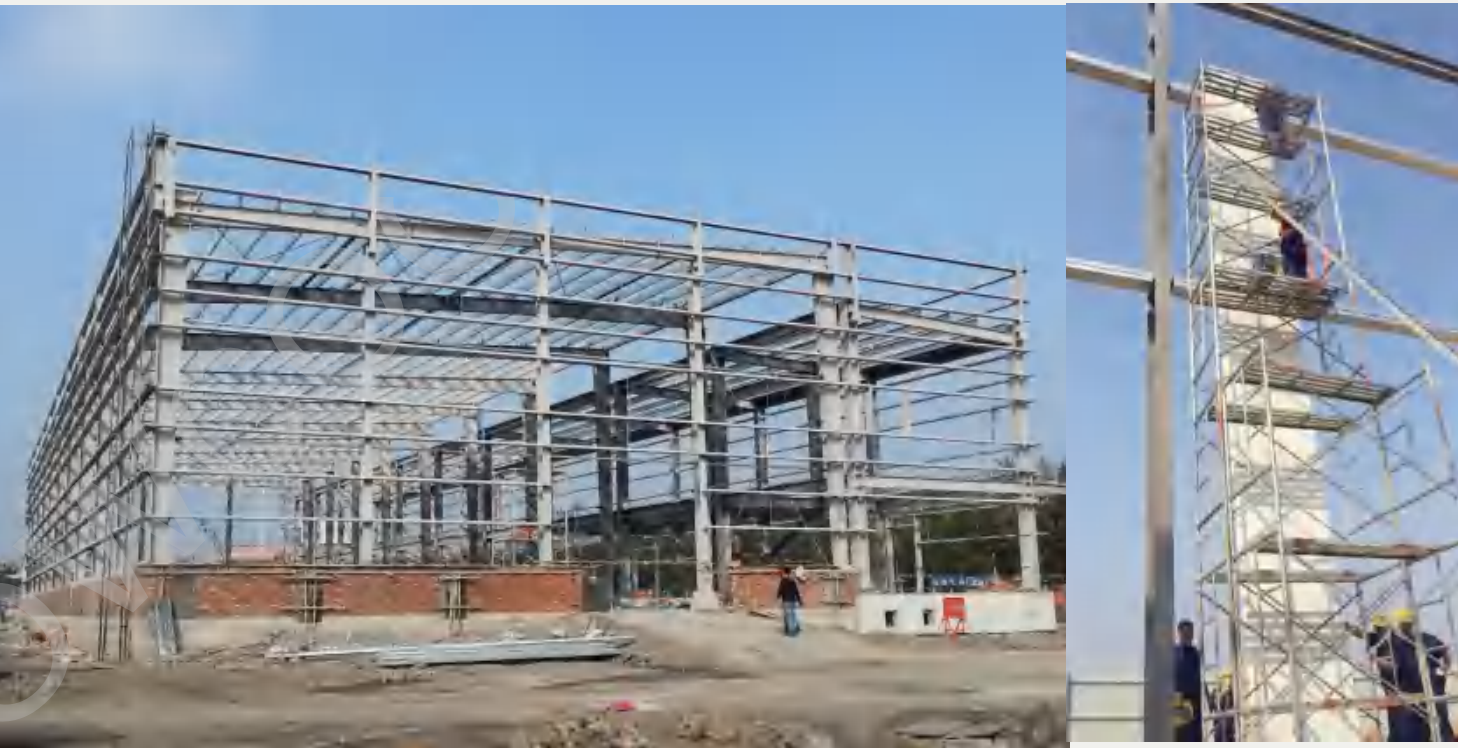
Main body of steel structure
