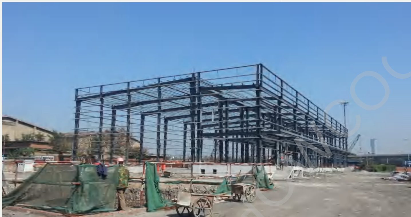
Main structure of large steel cold storage
