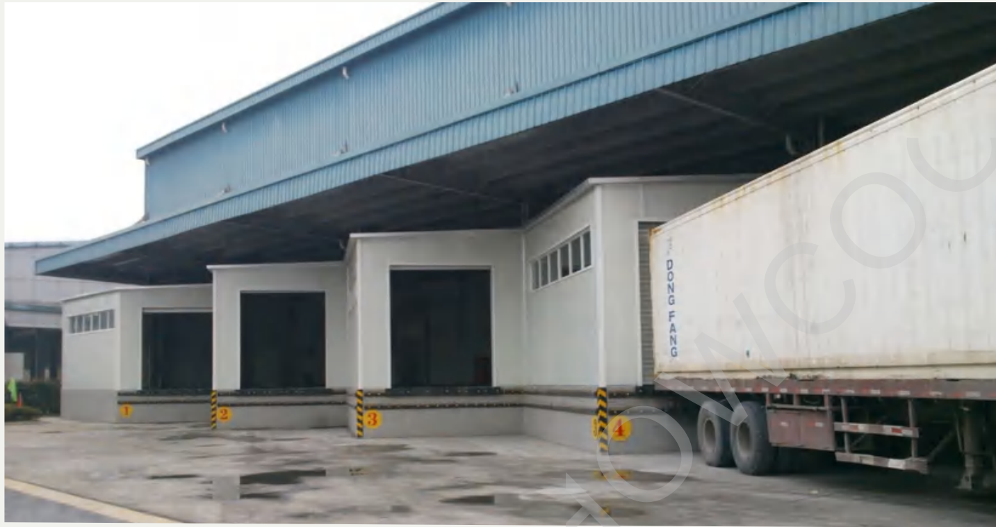
E-Commerce Distribution Center At Beijing
