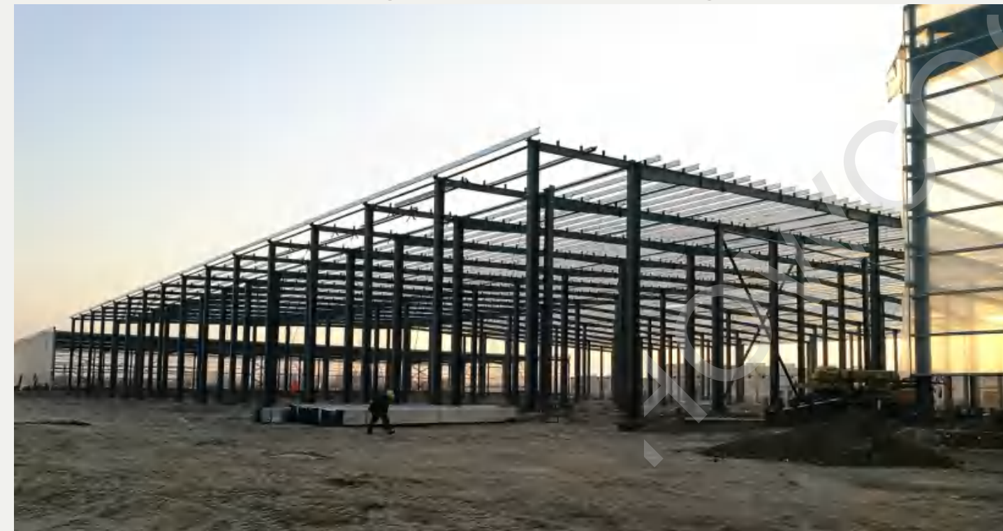
Main structure of large steel cold storage
