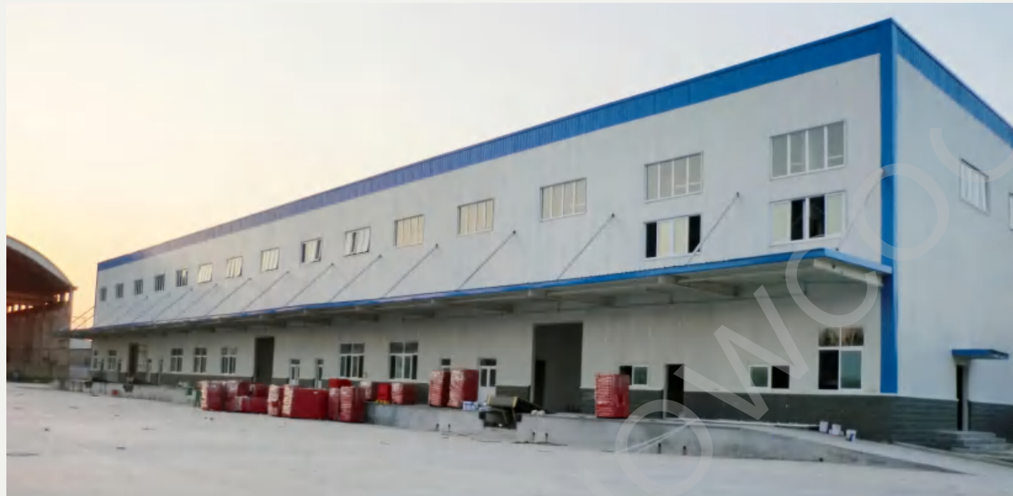
50000 m3 cold storage project
