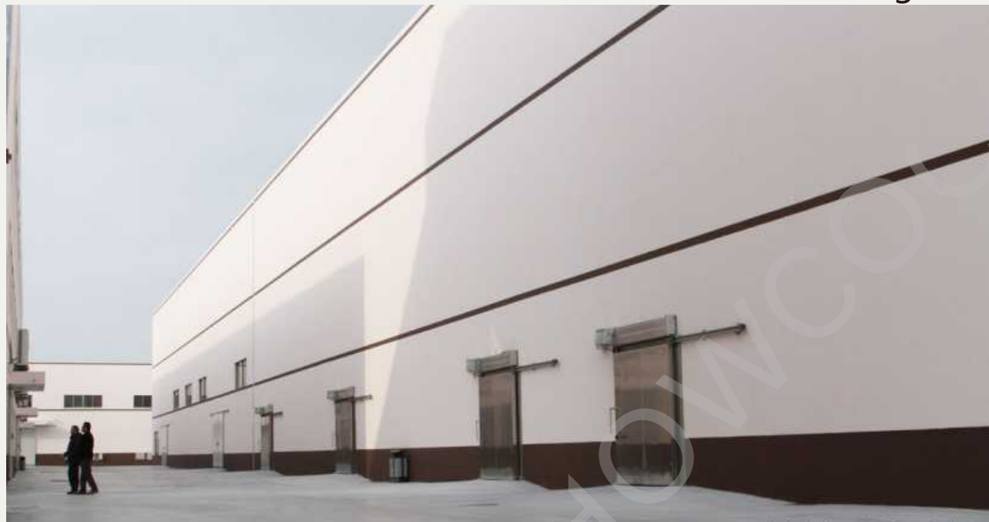
50000 cubic meters of e-commerce food cold storage
