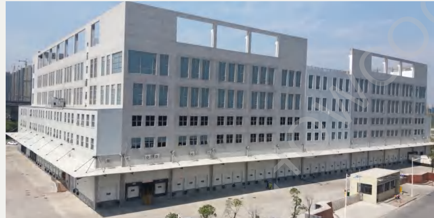
20000 tons cold chain logistics cold storage project
