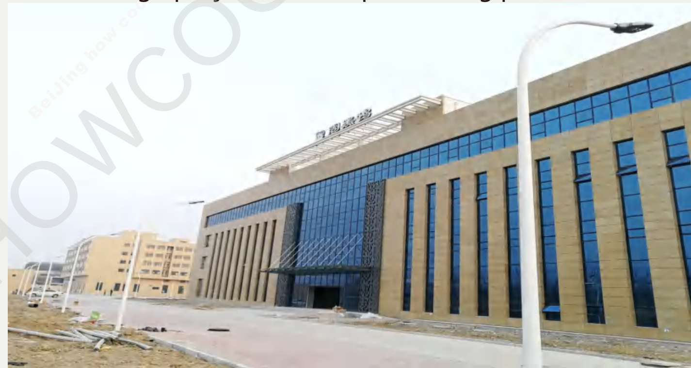
Cold storage project of food processing plant
