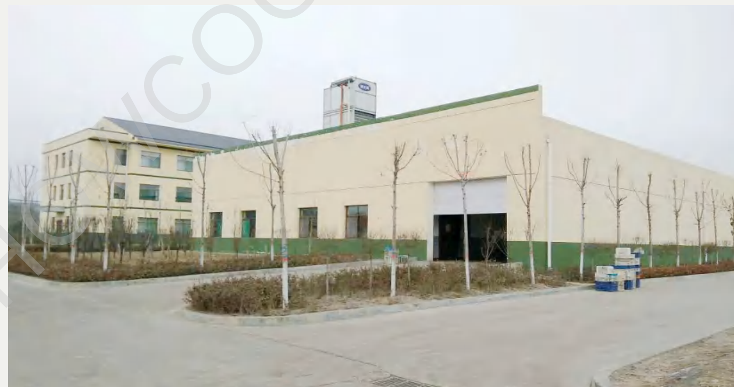
Cold storage of agricultural products logistics center
