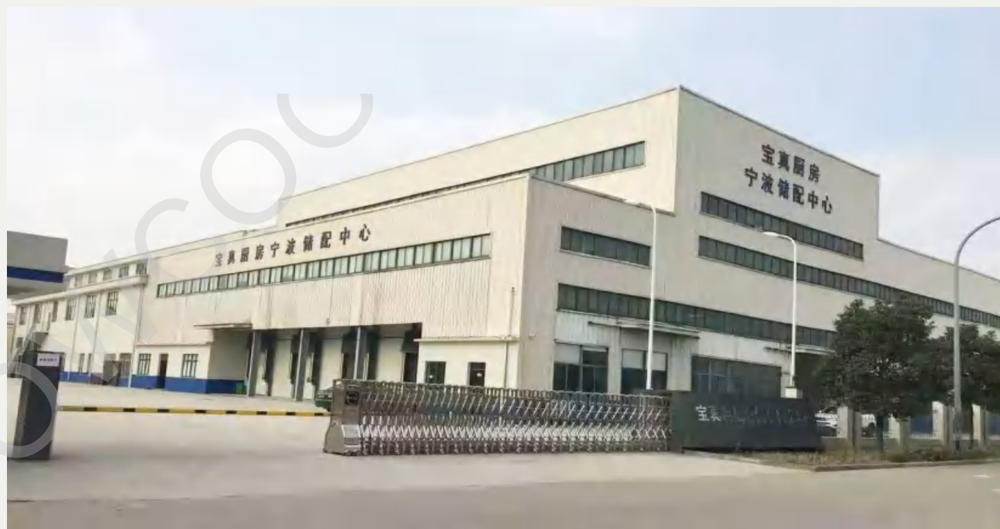
Cold storage project of central kitchen
