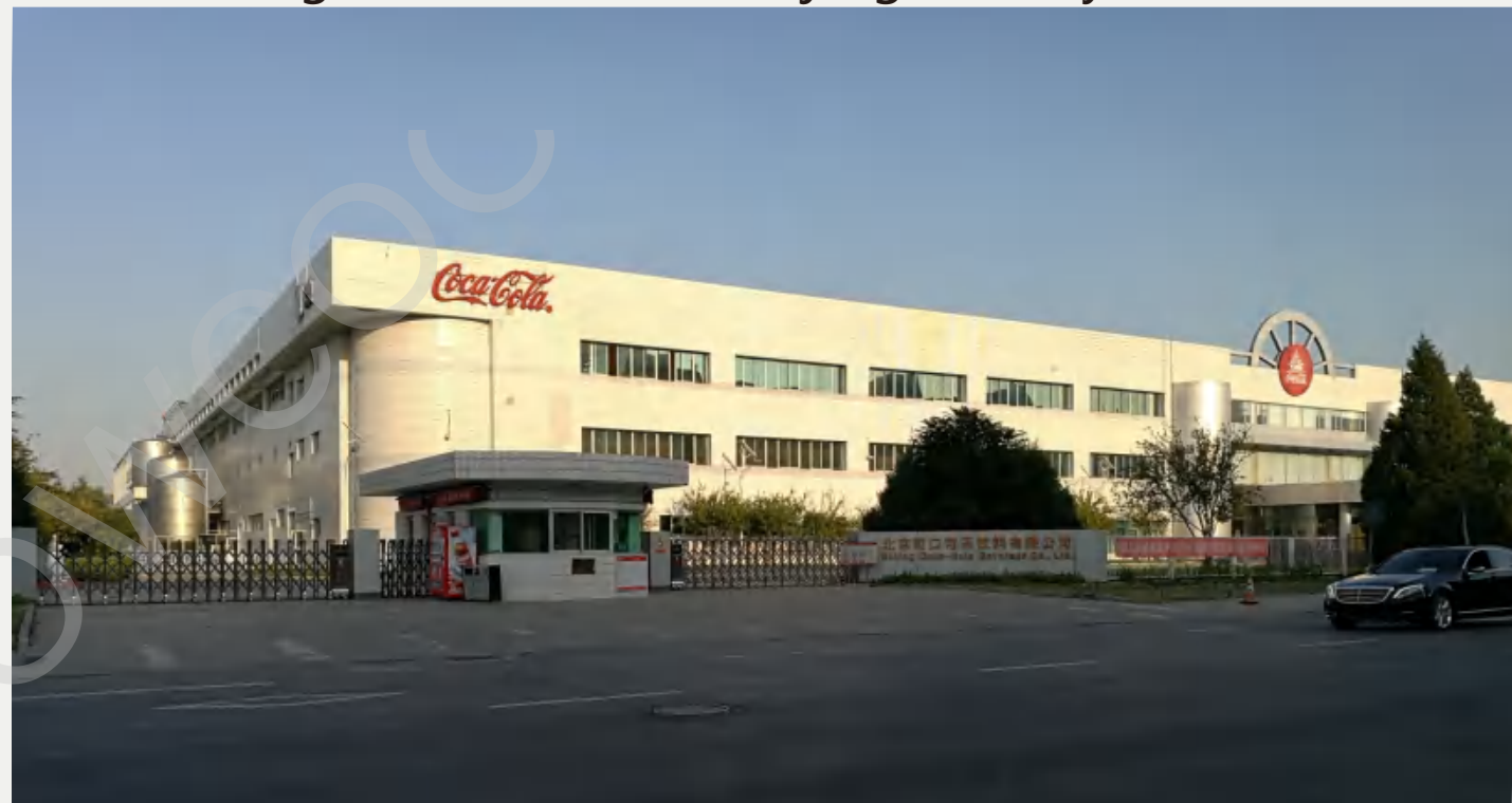
Cold storage of Coca Cola Beijing factory
