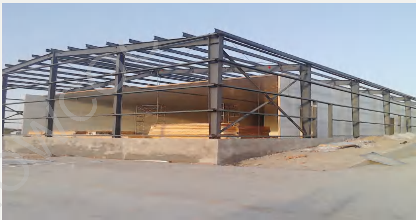
Main structure of large steel cold storage
