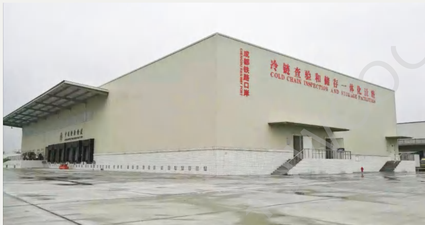
5000 ton cold storage project at railway port
