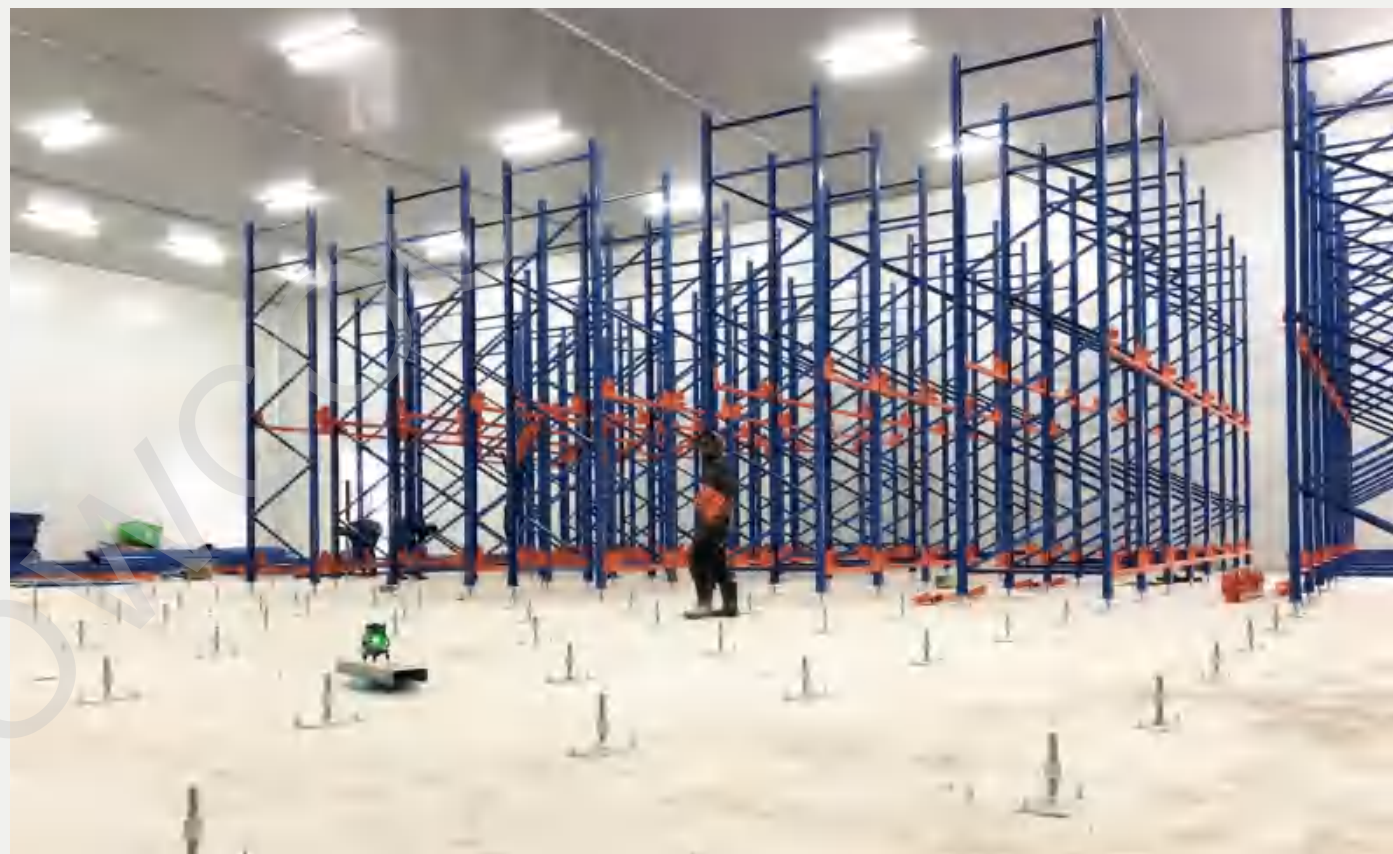
Shuttle Rack Installation
