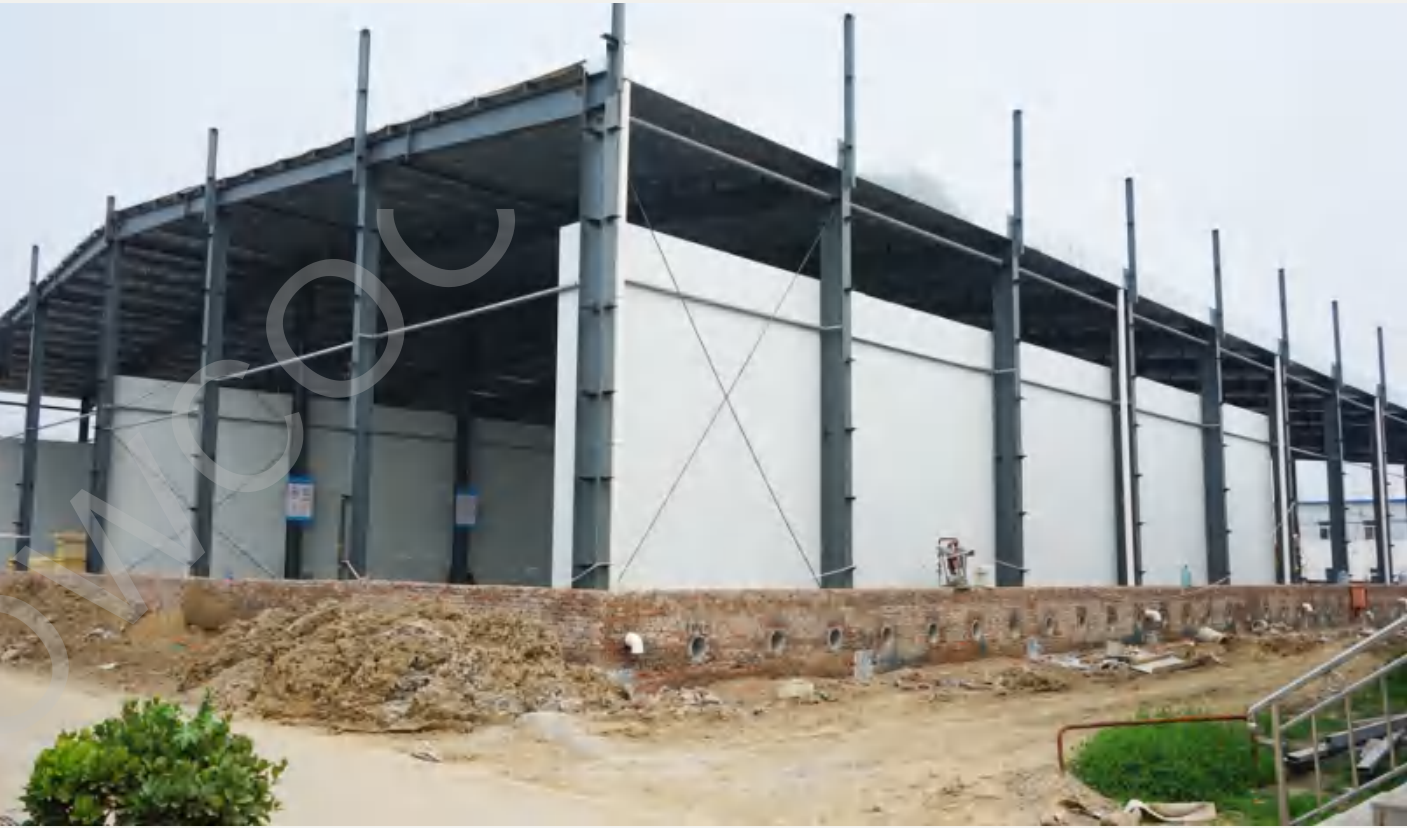
Building structure installation
